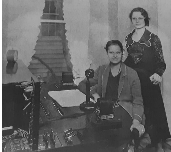
Kay & Viola Saunders at Jones home switchboard
